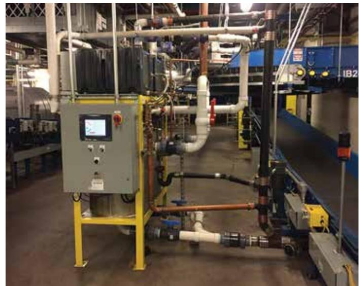
Unlike gravity plumbing, vacuum waste lines don't require continuous slope – they can go straight up, over or around any obstacle. Moving a sink from one wall to another becomes an easy, overnight job.
