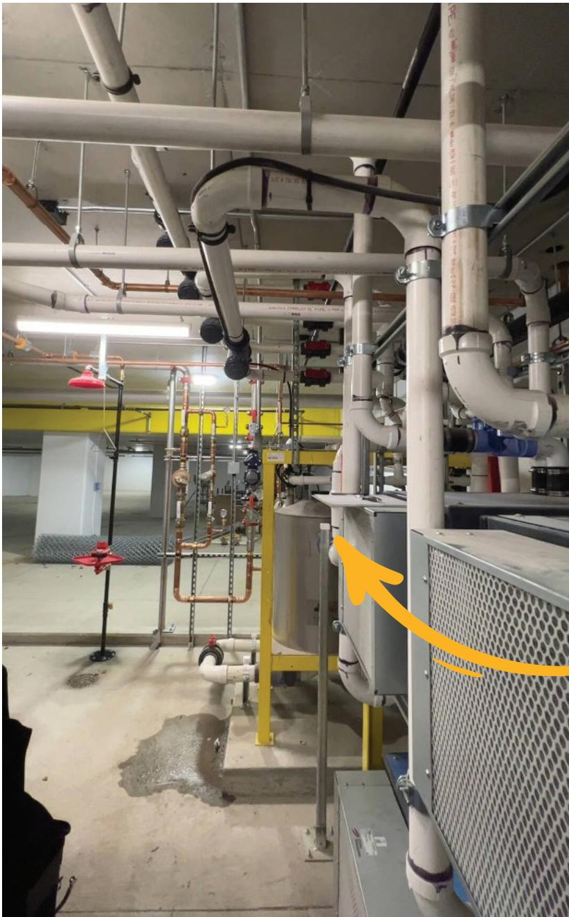
By installing the water-saving Acorn-Vac® vacuum plumbing system in its renovation of an historic office building, Holaday-Parks earned the building recognition for environmental sustainability. The building's AcornVac mid-level waste collection tank captures waste from upper-floor fixtures; here, it is supported by a framework (see the yellow bar).
